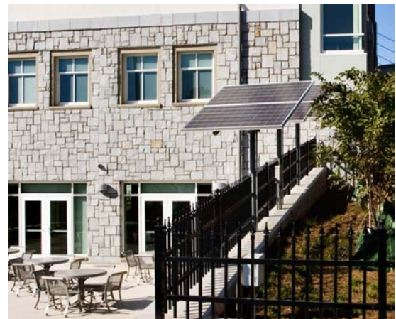
FIGURE 11. Solar Panels adjacent to a terrace power the pumps for the rainwater harvesting system (credit Ayers/Saint/Gross).
