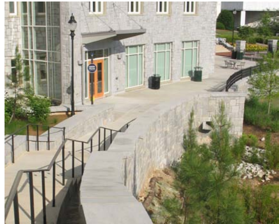
FIGURE 8. Stone weir conducts stormwater into the bioswale (credit Ayers/Saint/Gross).
