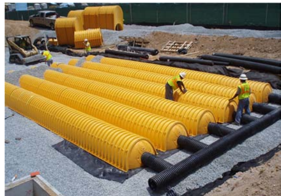
FIGURE 9. Stormtech chambers being placed below the swale during construction (credit Emory Photography).
