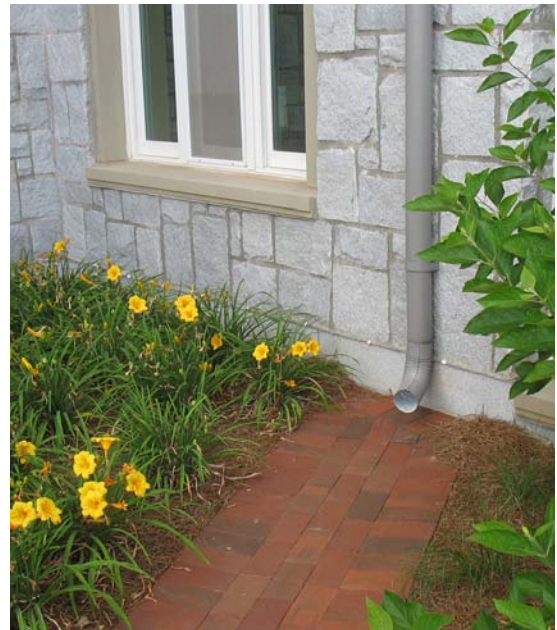
FIGURE 7. Downspouts spill to brick runnels in the landscape (credit Ayers/Saint/Gross).
