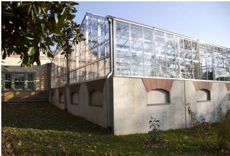
FIGURE 6. The simple gabled roof form and the standard two-foot glass module provided a modestly scaled greenhouse component. An additional bay or module can be easily added to expand the greenhouse without disruption to the established building scale. Photo Credit: Jessica Fogle of Archer & Buchanan Architecture, Ltd.
