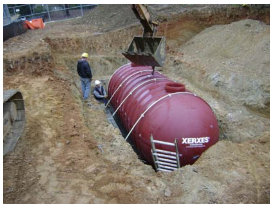
FIGURE 8. The 7,000 gallon rainwater harvesting tank being lowered in place. There is a lot below ground that one does not see or perceive is there. Photo Credit: Michael Bonacci, W.S. Cumby, Inc.
