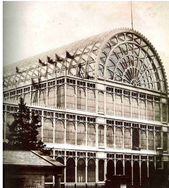
FIGURE 2. In Sir Joseph Paxton's Crystal Palace (1851) the repetition module of glass and structure provides scale, character, and style. Photo/Publication Credit: The Glasshouse by John Dixon, Phaidon Press Ltd., London/New York 1996, Pg. 5.
