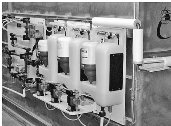
FIGURES 9 AND 10. Solid and liquid chemical inhibitor and biocide feed, monitoring, and control.
