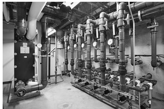
FIGURE 5. Well Manifold Piping and Heat Exchanger. (Paul S. Bartholomew Photography)
