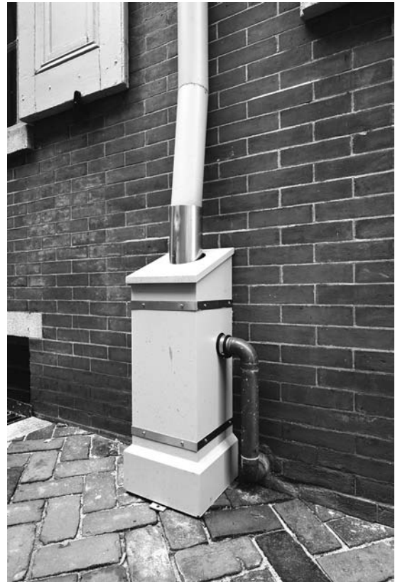
FIGURE 12. Diverter on Rainwater Conductor. (Paul S. Bartholomew Photography)
