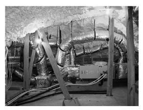
not being a moisture barrier, should not increase the likelihood of dry or wet rot in the rafters. We partnered with Energy Efficient Insulation (EEI), a certified and experienced Icynene dealer and installer, who sprayed 5–7 inches of foam. EEI was meticulous in getting into all the tight angles and recesses of the complicated rafter assembly.
