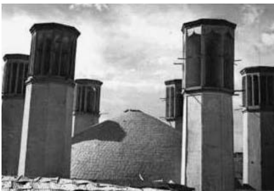
FIGURE 8A AND B. Cooling chimneys using evaporative cooling and the stacking effect of hot air: the Wind Towers of Yazd. Called 'Baadgeer', these wind catchers are characteristic of the central Iranian city of Yazd. As the name indicates the wind catchers were (and are) built to keep the buildings cooler during the hot and dry summers when the heat gets unbearable. The wind catchers are designed to catch even the smallest movement of air and direct it downwards to cool the living quarters below.
