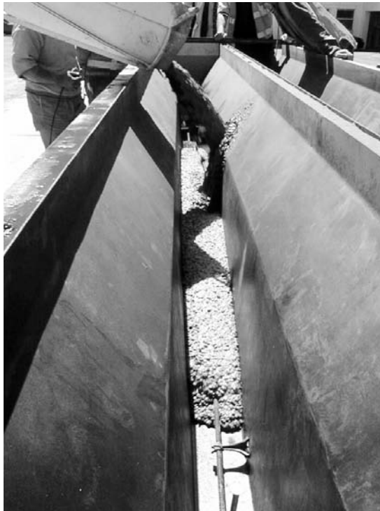
FIGURE 4. SCC allows more rapid and efficient precast concrete construction since no consolidation using vibration is required after casting.
