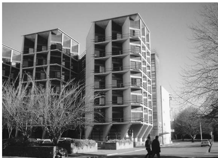
FIGURE 2. Computer Science Building at the University of Canterbury, Christchurch, New Zealand showing how concrete thermal mass is used to improve thermal efficiency.
