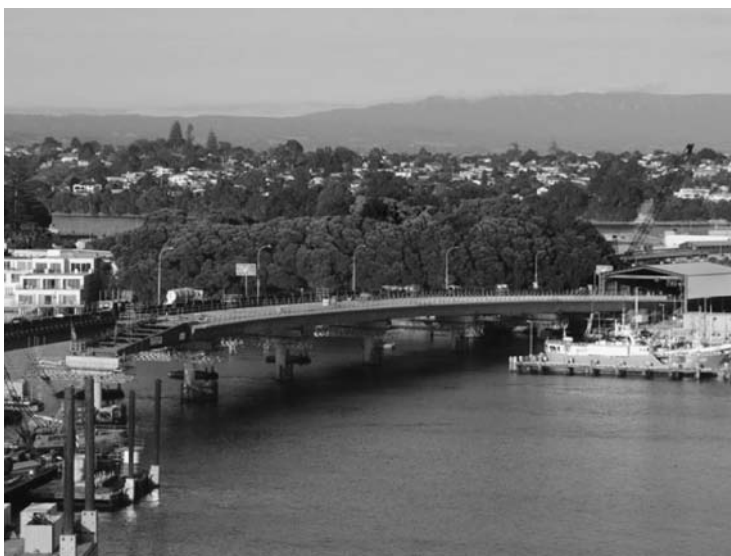
FIGURE 3. New Tauranga Bridge in New Zealand built over the harbour using an incrementally launched bridge deck system (Fletcher Construction).
