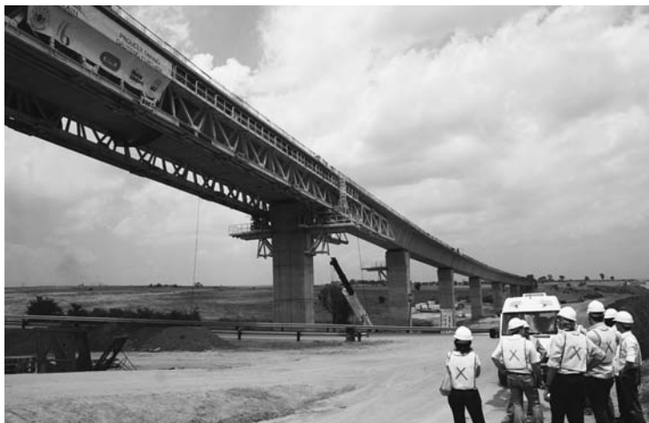
FIGURE 5. New concrete bridge for the Gautrain railway system in South Africa designed for a service life of 100 years.
