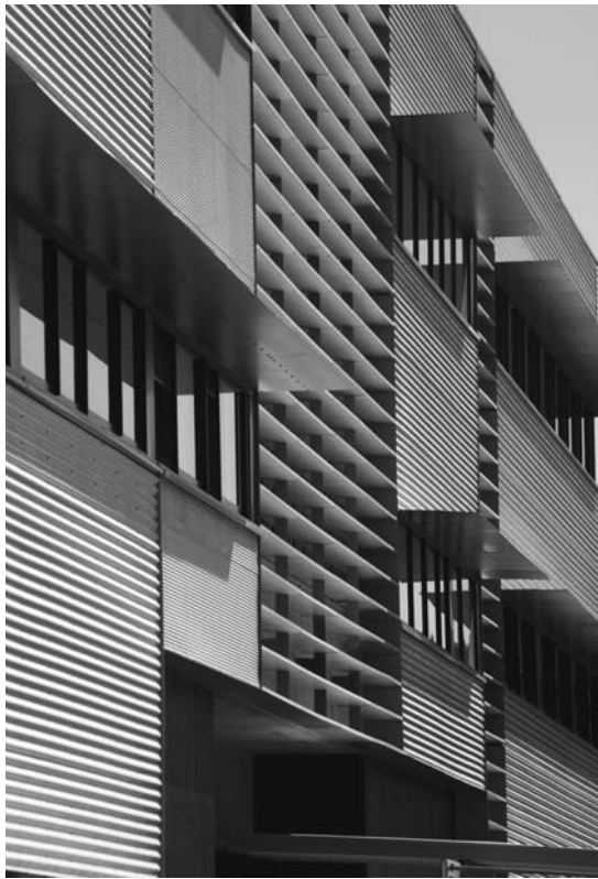
FIGURE 13. North facing façade indicating lightweight cladding, sun shading, and louvre system to stairs.
