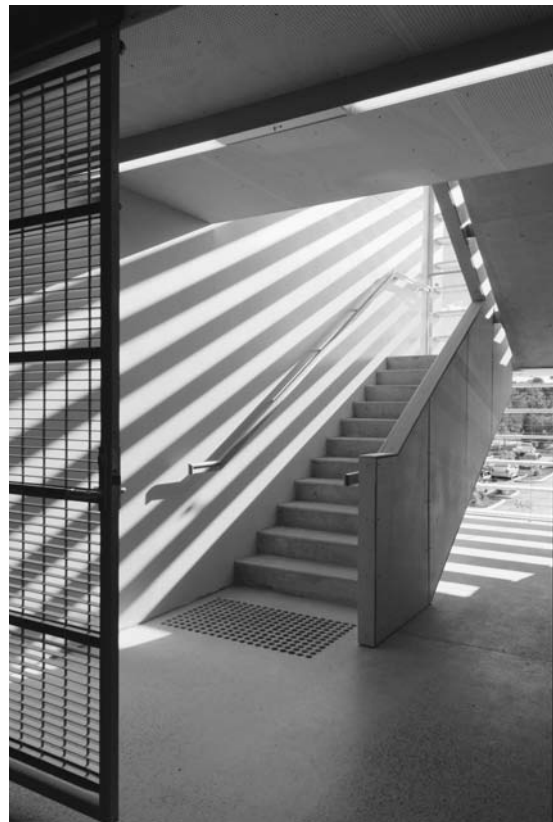
FIGURE 12. Typical naturally ventilated open stair.
