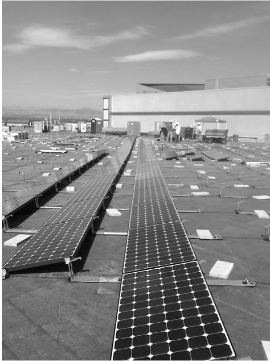
FIGURE 9. Solar Array Installation on CCC Roof.
