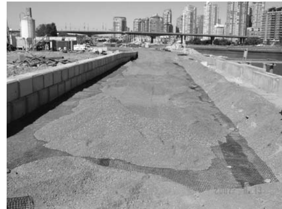
Southeast False Creek Silva Cell Installation
