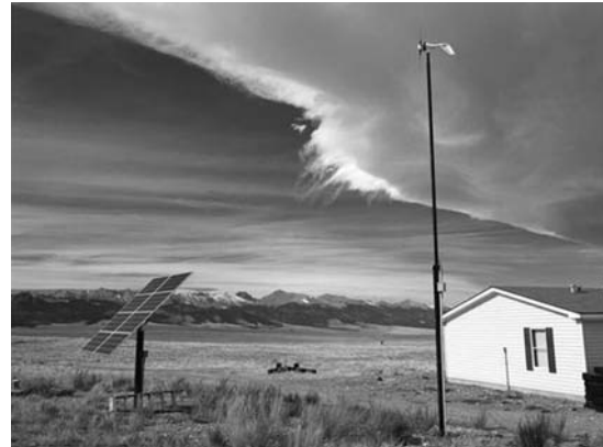
Southwest Windpower Air403, Colorado
