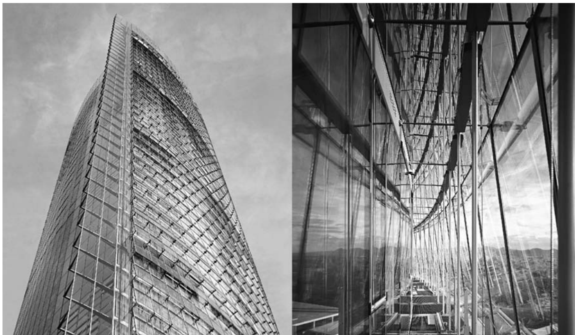
FIGURE 12. Post tower with advanced integrated facade for natural ventilation (2003; Fenn 2003).
