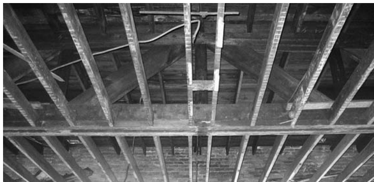
FIGURE 16. Detail of existing cypress box truss, ceiling joists, roof joists, and roof decking.
