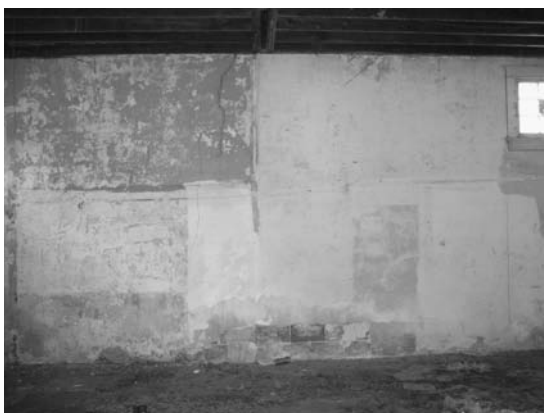
FIGURE 12. Existing load bearing wall with original plaster (note exposed structural tile in lower middle portion of photograph at floor).
