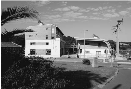
FIGURE 2. Jubilee Wharf, Penryn, UK (2006). This zero energy development uses 4 micro turbines to provide power. Evacuated tubes provide solar hot water. The roof has been designed for PV, but no PV is presently installed. Directional wind cowls assist with natural ventilation to the point that no A/C is provided. A 75kW wood pellet boiler provides under floor radiant heating. The building is super insulated with 300mm of insulation netting a U value of 0.1\text{W/m}^2/\text{°k} . Designed by ZEDFactory.
