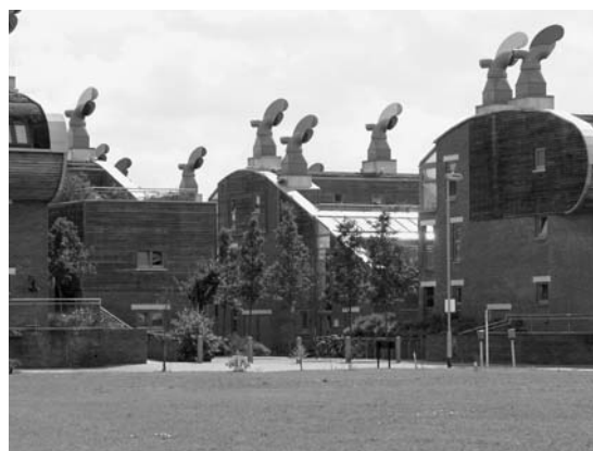
FIGURE 1. Beddington Zero Energy Development (2002). This project takes a holistic approach to energy reductions. It uses a combined heat and power plant to provide energy to the complex. Energy requirements are reduced through passive solar heating strategies. The project uses super insulation to assist with heat retention. Air conditioning is not provided. Wind cowls assist with natural ventilation for cooling. Designed by ZEDfactory.
