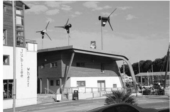
FIGURE 2. Jubilee Wharf, Penryn, UK (2006). This zero energy development uses 4 micro turbines to provide power. Evacuated tubes provide solar hot water. The roof has been designed for PV, but no PV is presently installed. Directional wind cowls assist with natural ventilation to the point that no A/C is provided. A 75kW wood pellet boiler provides under floor radiant heating. The building is super insulated with 300mm of insulation netting a U value of 0.1\text{W/m}^2/\text{°k} . Designed by ZEDFactory.
