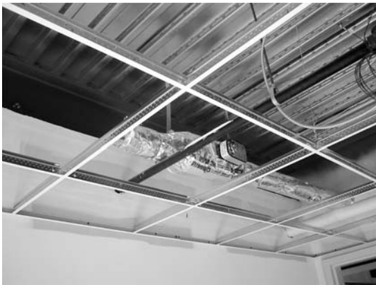
FIGURE 7. Ventilation air control assembly.
