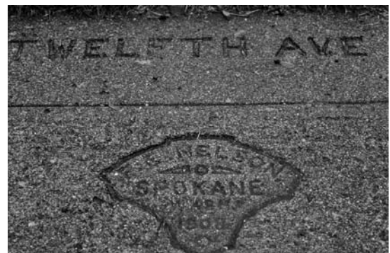
FIGURE 6. “F. E. Nelson Spokane, Wash. 1908”—An example of old concrete pavement with no maintenance in 100 years.
