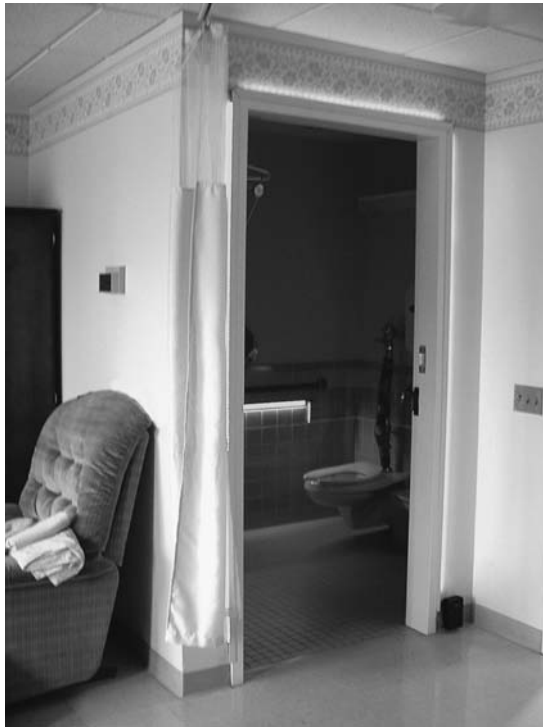
FIGURE 6. Nightlights with motion sensor control provide dim illumination to the local environment as well as enhanced spatial perceptual information by providing horizontal and vertical cues, but only when needed by the occupant.
