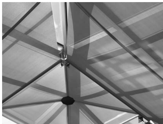
FIGURE 13. Greenhouse Shading. The greenhouse, at the top of the lightwell, was equipped with retractable shade cloths that were deployed on all, or all but the NW quadrant, throughout the study.
