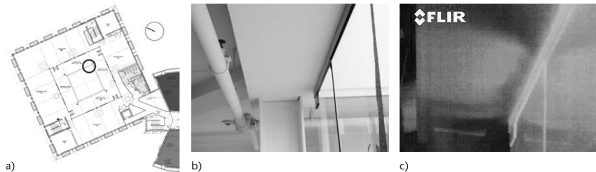
FIGURE 11. Greenhouse Door. The greenhouse on Level 4 possessed an unsealed glass door on the northwest side (a, b), allowing warm air to enter, as viewed against the adjacent soffit (b, c). Airspeed mode: 140fpm; maximum: >400fpm; entry air temperature: 87.2°F; ambient air temperature: 74.5°F. (8/21/07, 11:36 a.m.).
