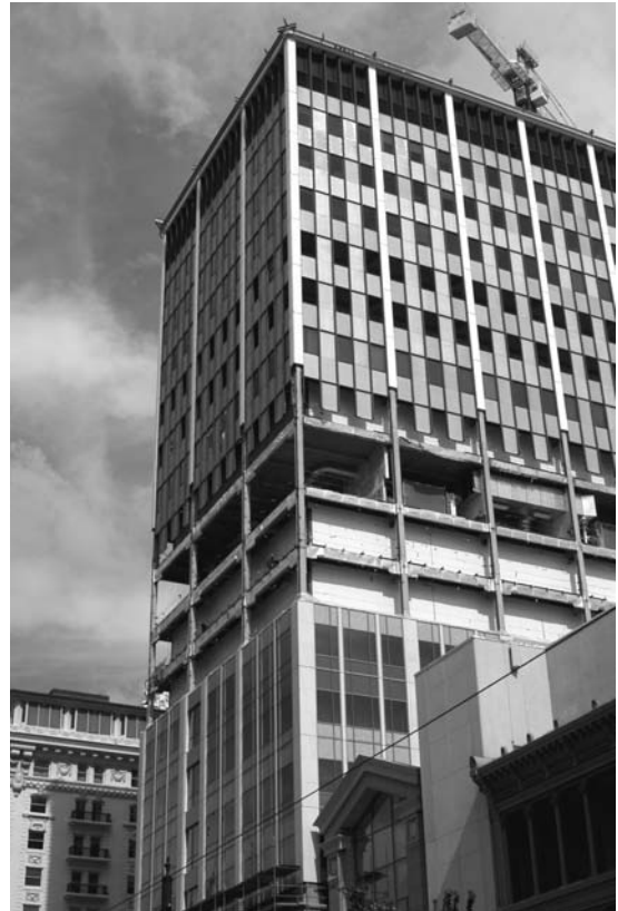
FIGURE 2. Technology of the twenty-first century can be used to reclad mid-twentieth-century façades that have become aesthetically “dated” with more contemporary facades. In some instances, this is done to update the appearance while in others it has been done to reduce operating and maintenance costs (© 2005, Robert A. Young, all rights reserved).
