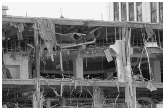
FIGURE 4. Without any substantial network of recycling options in place, demolition of existing buildings creates increasingly greater pressures on landfill space. Similarly, the complete replacement of an existing building with a new building of equal or greater size continues the cycle of extraction of raw materials to create new building products (© 2007, Robert A. Young, all rights reserved).
