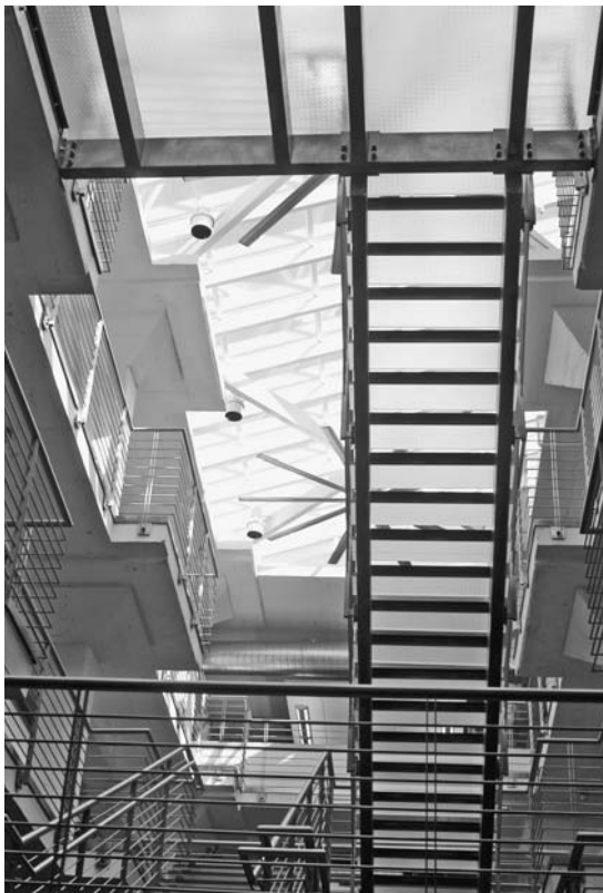
FIGURE 11. The large atrium created by removing sections of concrete slab provides light and air flow paths that enhance the energy performance of the building (©2008, Robert A. Young, all rights reserved).
