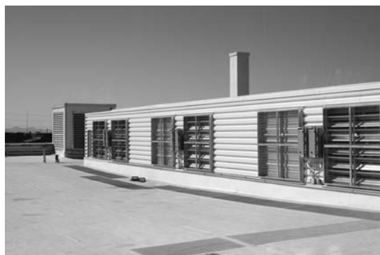
FIGURE 8. Lighter colored roofing reflects solar energy and helps to reduce internal heat gain and the urban heat island effect (©2008, Robert A. Young, all rights reserved).
