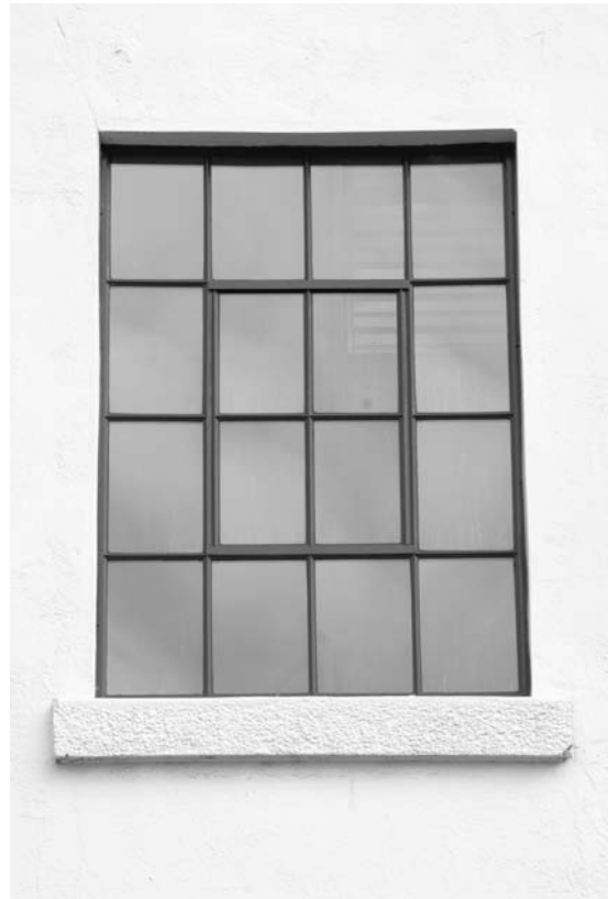
FIGURE 5. The single pane glazing in the original industrial sash was replaced with laminated glass to enhance the energy performance of the windows at the Big-D Construction Office. This allowed the window rehabilitation to retain its original appearance and thus conform to the Secretary of the Interior Standards for Rehabilitation (© 2007, Robert A. Young, all rights reserved).
