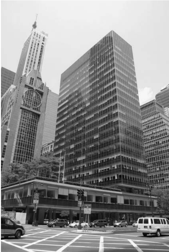
FIGURE 3. By the late-twentieth century, the curtain wall system on the Lever House, completed in 1952, had fallen into disrepair. The curtain wall was removed and an entirely new curtain wall system was installed to upgrade the appearance and energy performance of the building (© 2007, Robert A. Young, all rights reserved).
