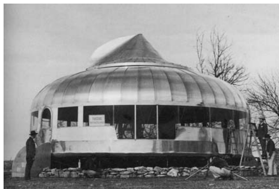
FIGURE 1. The Dymaxion (Wichita) House at the construction site, upon finishing the outer shell. (Source [5])
