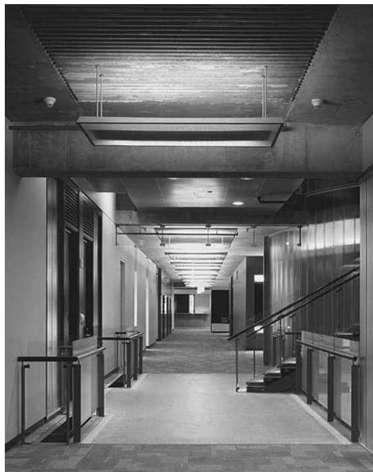
FIGURE 6. Bahen Centre, University of Toronto. Exposed Slab Soffits with Cast-in-place Corrugations.
