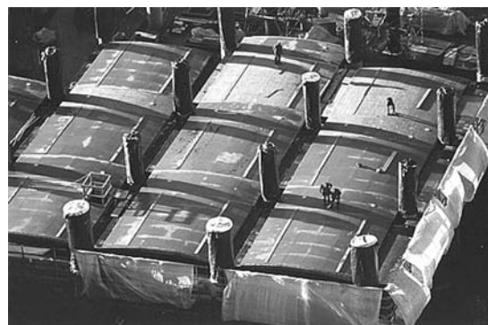
FIGURE 4. Library Square, Vancouver. Concrete Formwork for Exposed Barrel Vault Ceiling.
