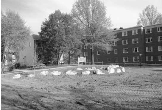
FIGURE 7. Fine grading at the University of Delaware rain garden.
