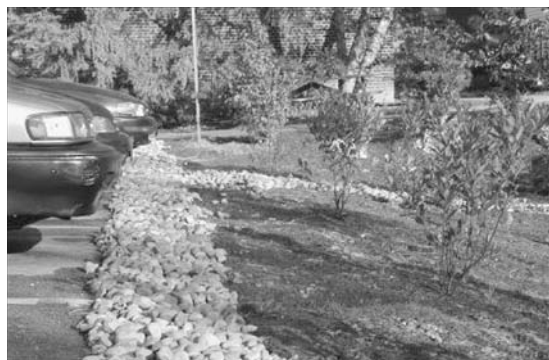
FIGURE 10. Installation of cobble erosion control filter strip.
