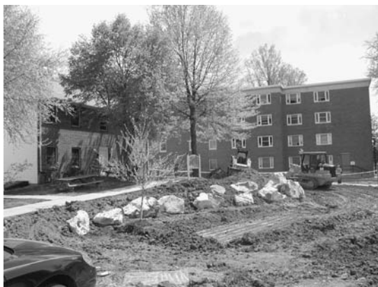
FIGURE 6. Earthwork and excavation at the University of Delaware rain garden.
