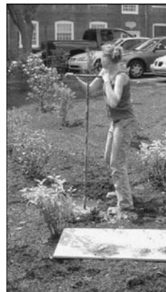
FIGURE 11. Performing soil borings to install pea gravel drains through clay layer.
