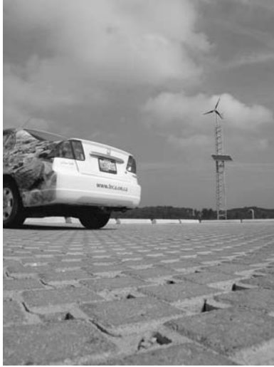
FIGURE 4. Permeable pavement installation at Seneca College, King Campus, Ontario. (Photo courtesy of Toronto and Region Conservation Authority.)
