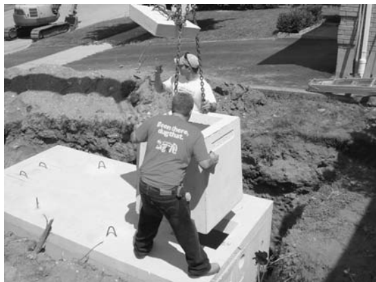
FIGURE 10. Installation of concrete tank for rainwater harvesting system at a single family home, Guelph, Ontario. (Photo courtesy of Chris Despins, University of Guelph.)
