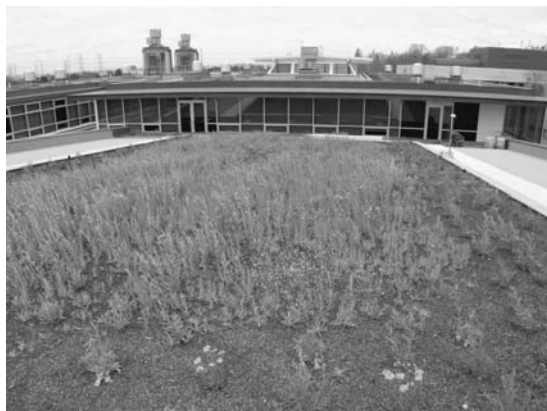
FIGURE 7. Extensive green roof with 10% slope at York University. (Photo courtesy of Toronto and Region Conservation Authority.)
