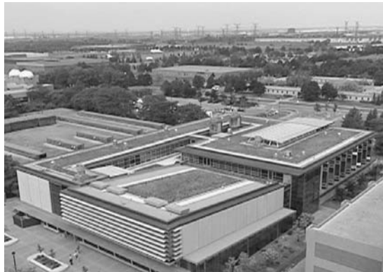
FIGURE 6. Extensive green roof at York University, Toronto, Ontario. (Photo courtesy of Toronto and Region Conservation Authority.)
