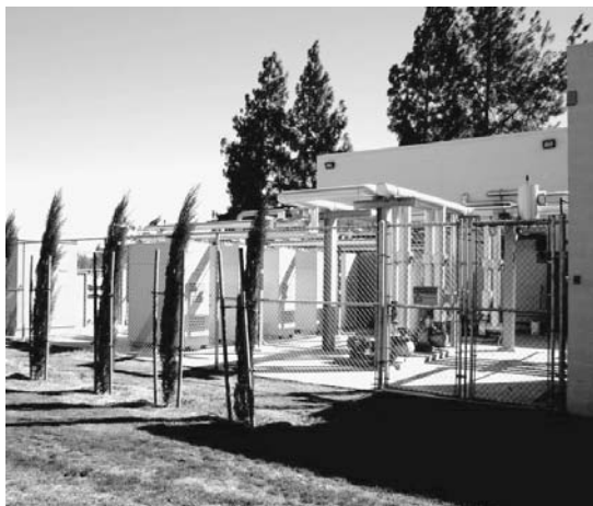
PHOTO 6. 360 kW cogen installation using six Capstone microturbine units in Woodland Hills, CA. Hot water byproduct loop connects to absorption chillers for air conditioning purposes. (Courtesy of Capstone Turbine Corp.)
