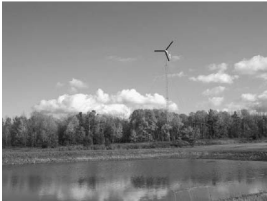
PHOTO 1. 10-kw wind turbine near Ithaca, NY, in summer. Turbine is mounted on 80' tower, which is held in place on three sides with guy wires. (Courtesy of Michael Miles.)
