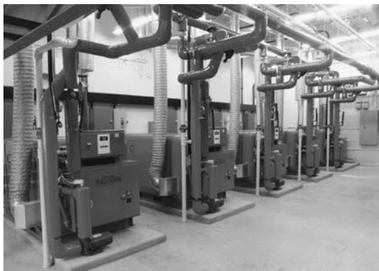
PHOTO 5. 375 kW cogen installation using five Tecogen reciprocating generator units in Waverley, NY. Piping loops (red) connect hot water byproduct to DHW, hydronic heaters, or absorption chillers. (Courtesy of Tecogen, Inc.)
