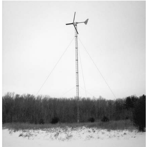
PHOTO 1A. 10-kw wind turbine near Ithaca, NY, in winter. Turbine is mounted on 80' tower, which is held in place on three sides with guy wires. Photograph was taken at around 3 P.M. on January 28, 2007. In a light breeze, rotations were fluctuating around 70 RPM and the output was around 0.5 kW. (Photograph from author's own collection.)
