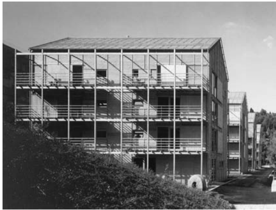
FIGURE 7. View of the four residential buildings facing the river (photo: C. Richters).
