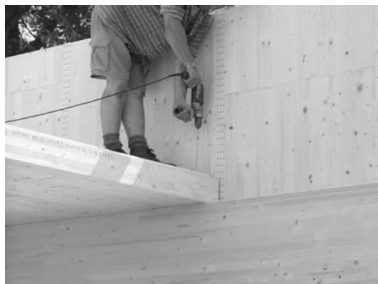
FIGURE 2. Assembly of prefabricated floor and wall panels on site (photo: FGH).
