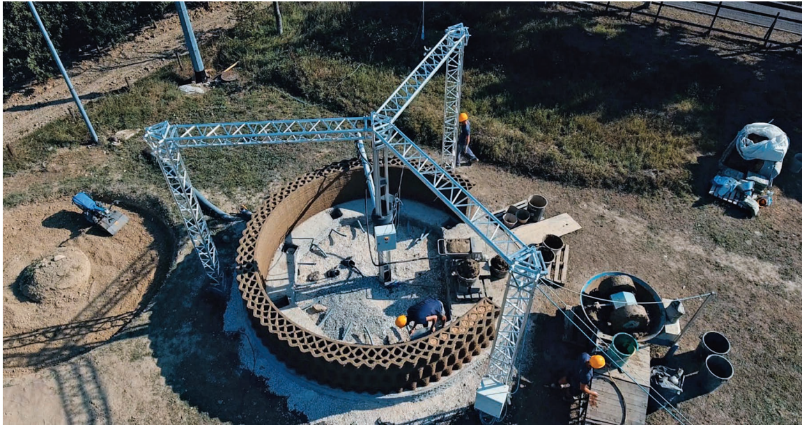
FIGURE 13. Gaia, the first 3DP structure made from earth, walls interior section view (Courtesy of Chiusoli 2018)
