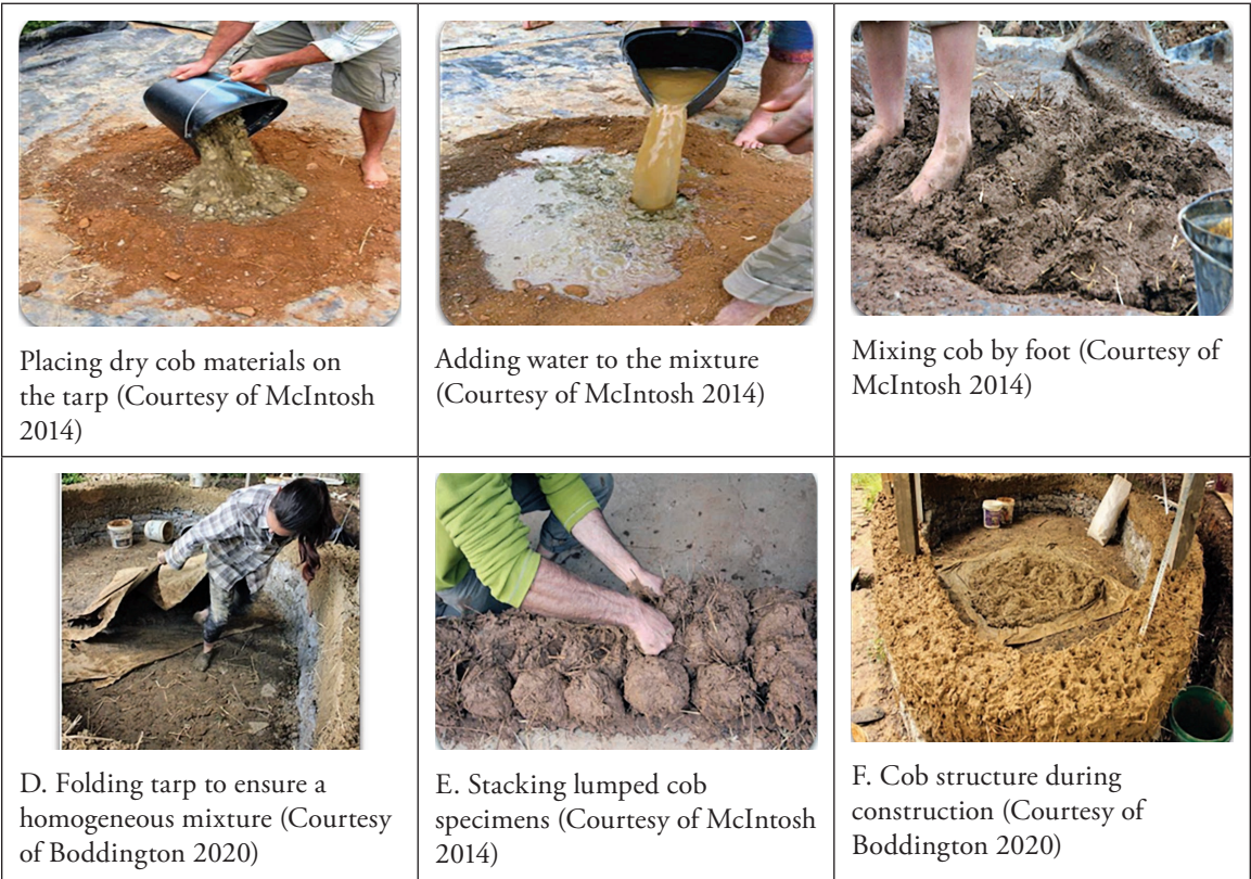
FIGURE 3. The traditional cob construction process.
