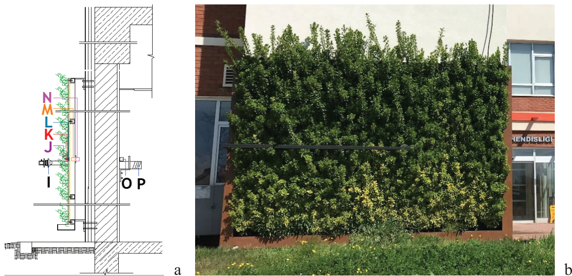
FIGURE 9A, B. Section of vegetated facade test assembly(left) and image of vegetated facade system (right).
