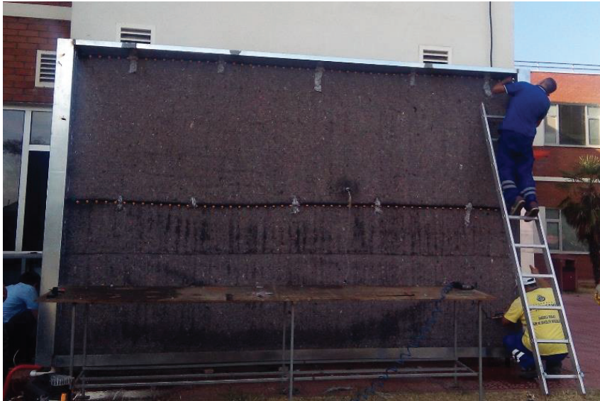
FIGURE 5. Geotextile felt material attached on PVC panel and irrigation pipes mounted on the felt layer (image of VFS before plant layer applied).
