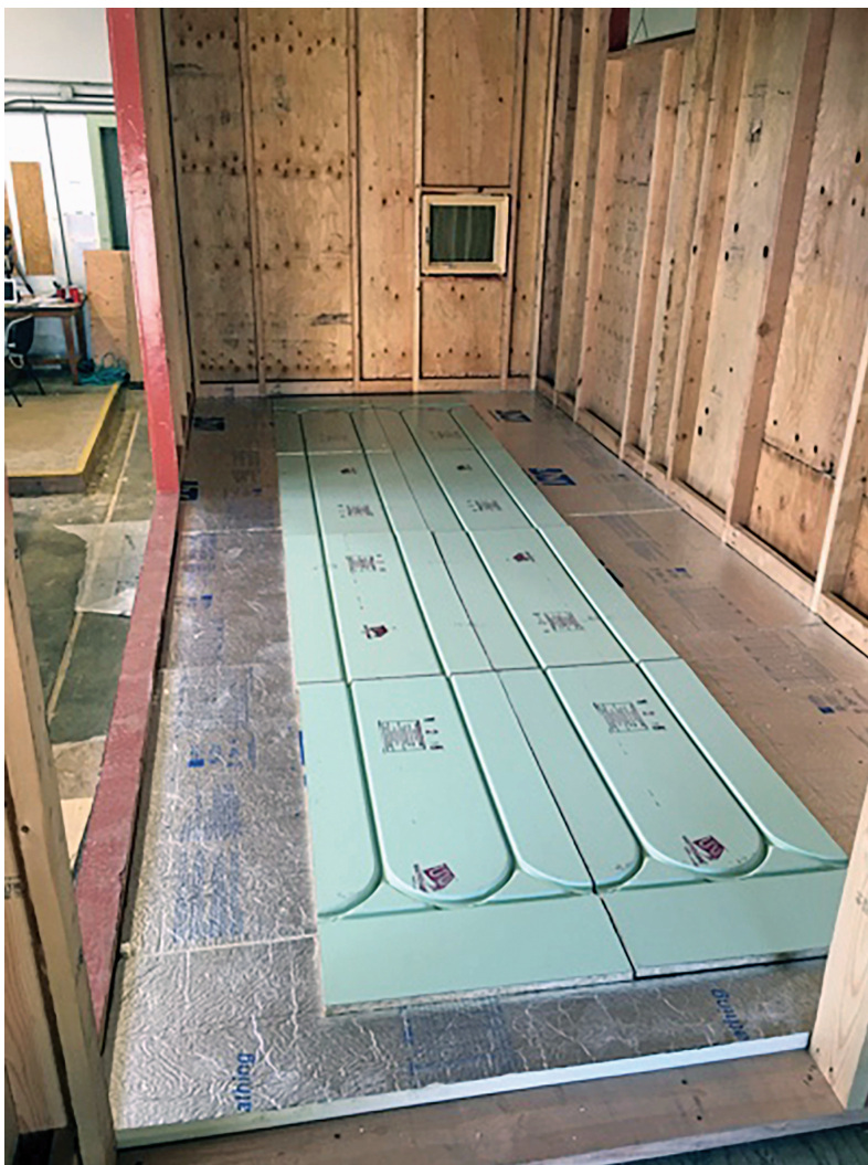
FIGURE 3. THIMBY Warmboard Radiant Floor Layout.
