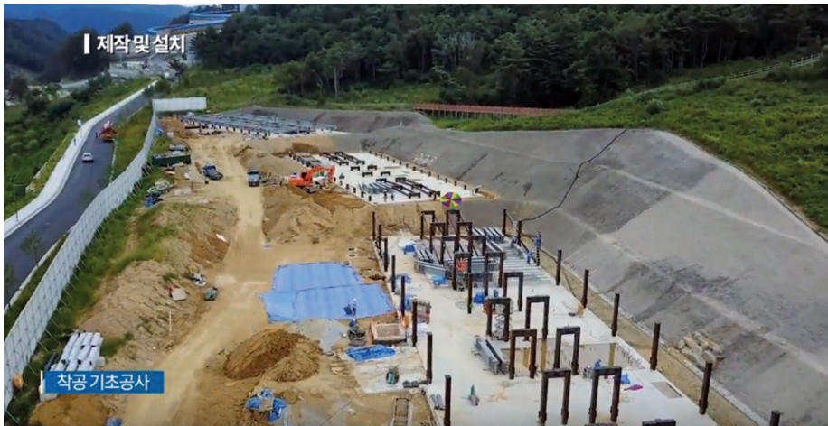
FIGURE 7. Piloti construction.
