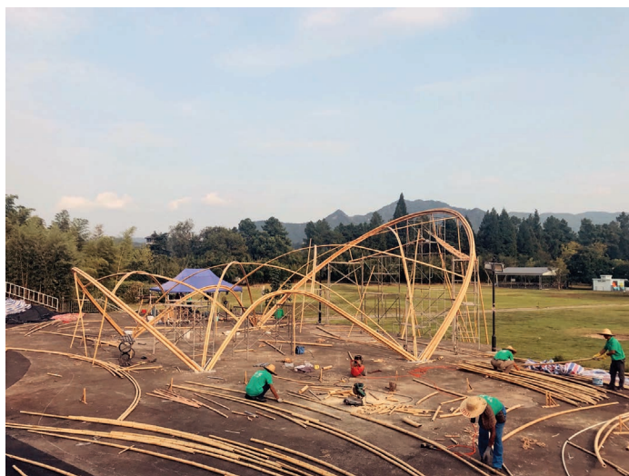
FIGURE 12. Installation process indicating the primary structure.
