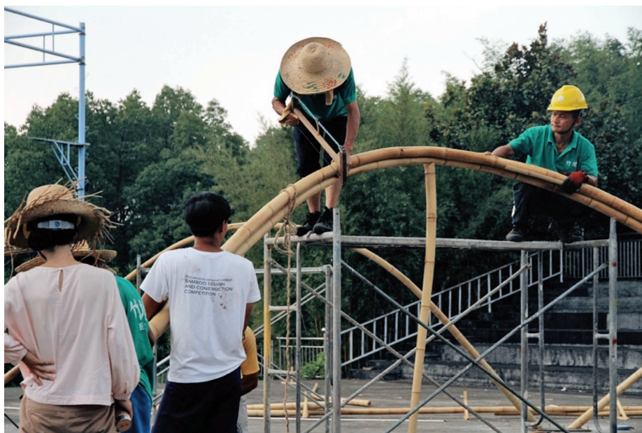
FIGURE 15. Onsite installation by matching corresponding pieces.
