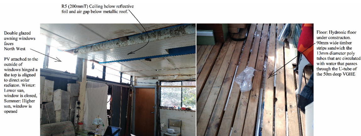
FIGURE 3. Double glazed windows with a PV panel on the north-west wall (Left) and the floor-HR with 13 mm poly pipes (Right).
