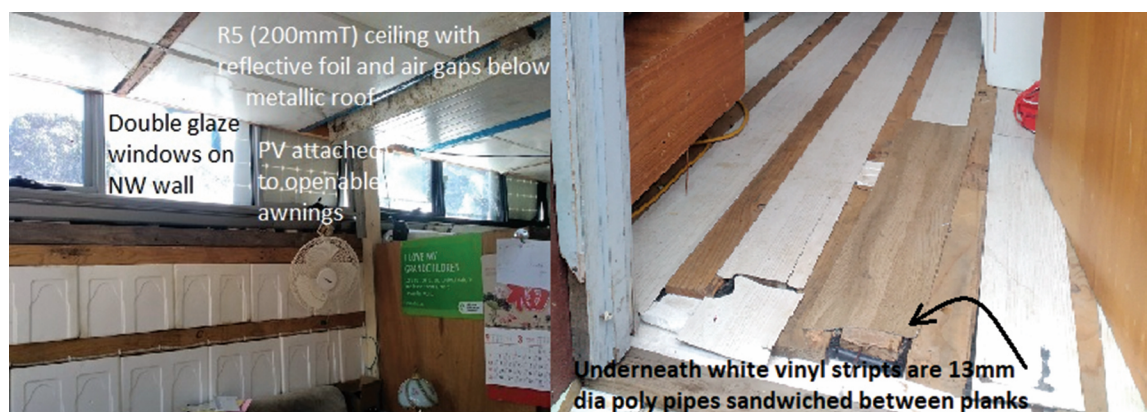
FIGURE 2 Internal building components of the experimental house constructed in Melbourne
