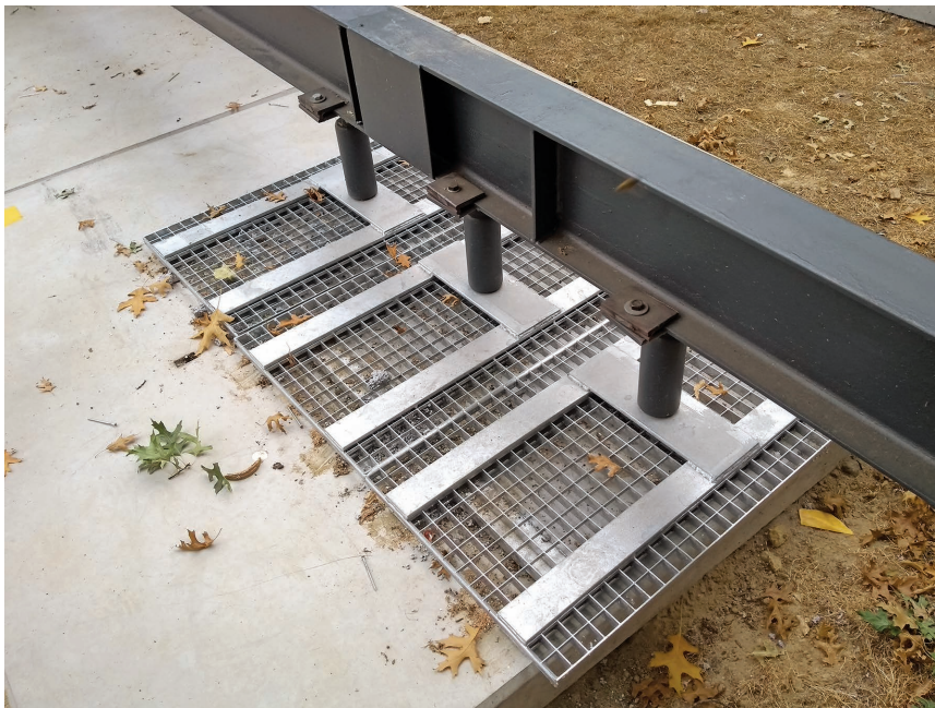
FIGURE 9. Steel footings in the TU/e. They were placed on the ground in Dubai.
