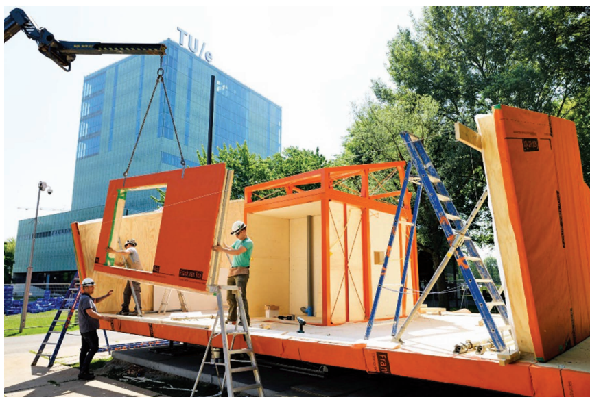
FIGURE 17. (Orange) foils stick out from the panels to seal them afterward (Team VIRTUe 2019).
