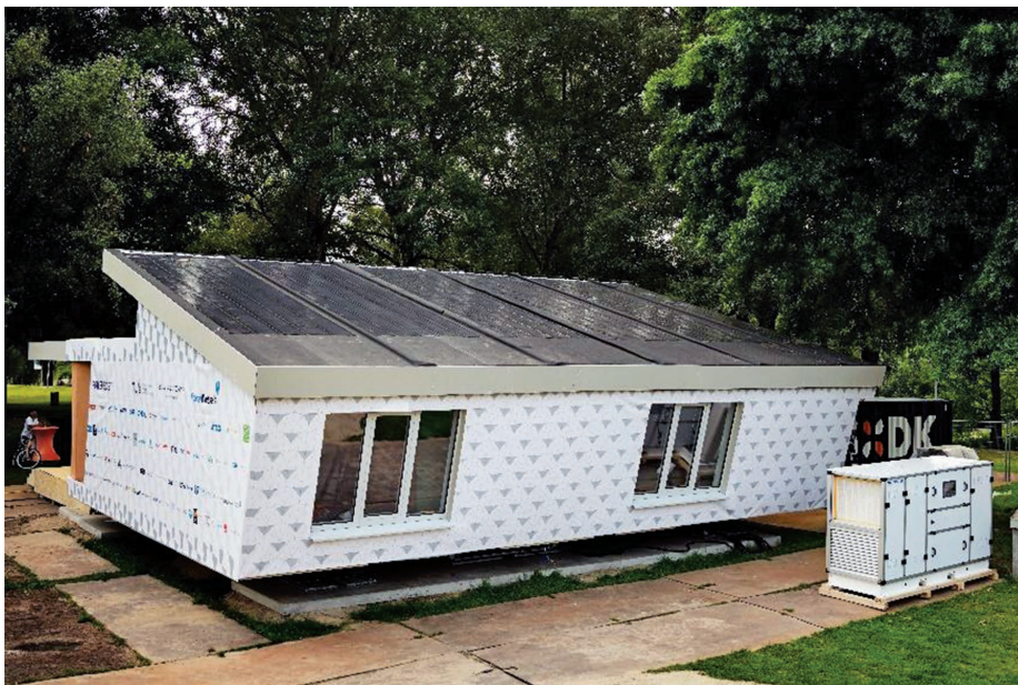
FIGURE 34. The building integrated photovoltaic-thermal system was integrated into the roof (Team VIRTUe 2019).
