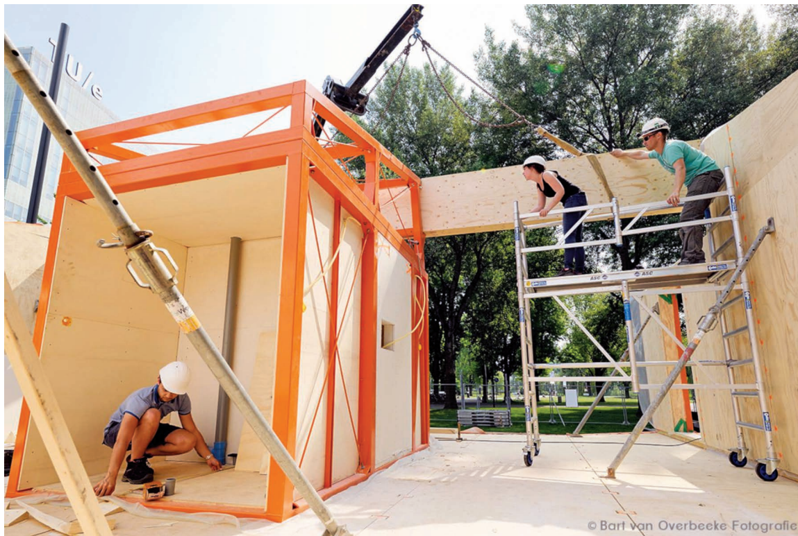
FIGURE 11. The roof module laid over the technical module (source: Bart van Overbeeke). The North beam laid over the roof module and exterior walls (Team VIRTUe 2019).
