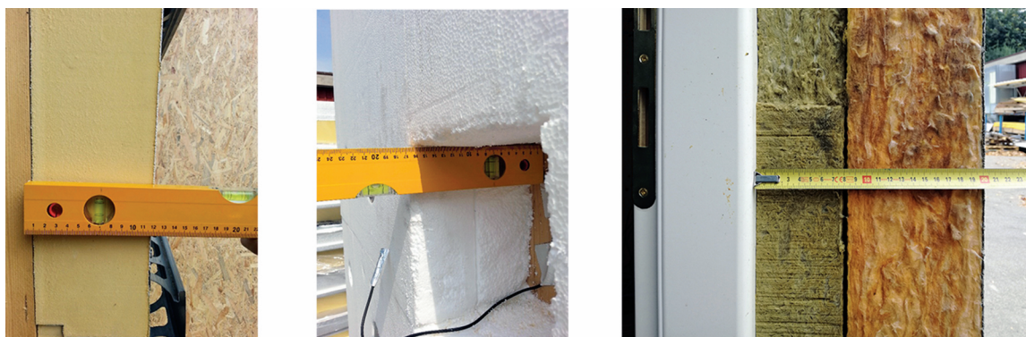
FIGURE 3. Zoom on thickens insulation during installation on the chambers. Left: Polyurethane foam Isotec® wall; Center: EPS panel; Right: double panel in high density rock wool.
