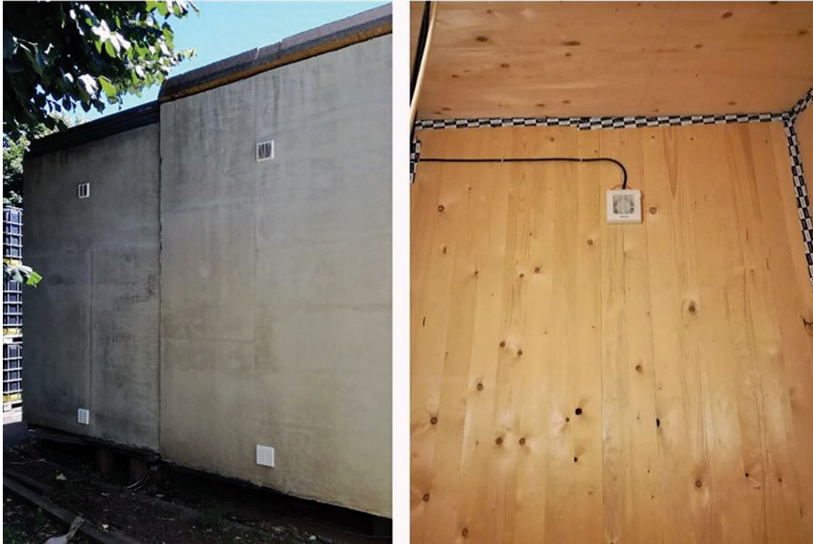
FIGURE 10. North façade of the text box. The white elements are the ventilation extract fans and the ventilation grilles.
