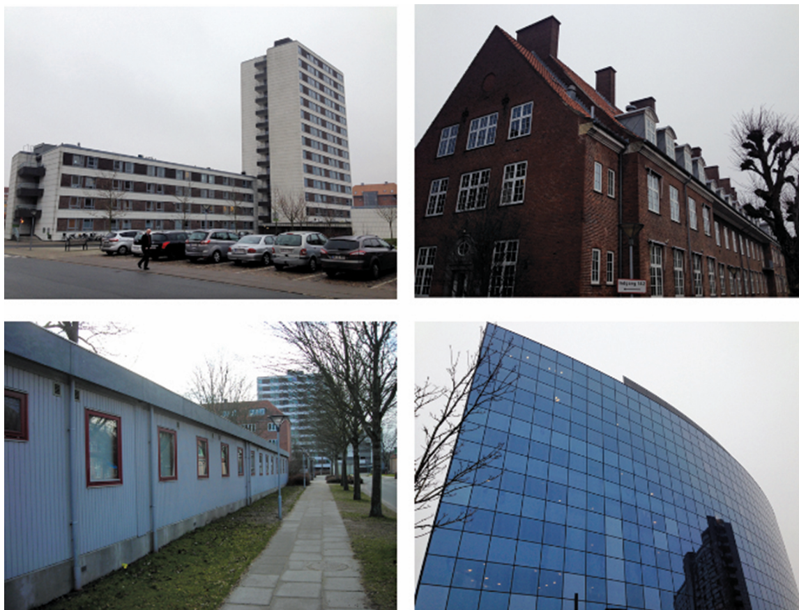
FIGURE 1. Examples on building types on site. Top left: Characteristic concrete building (Built 1960s-1970s). Top right: Red Masonry buildings (Built 1912). Bottom left: Barracks (Built 1980s). Bottom right: An example of newer steel construction (Built 2000s).
