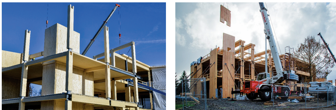
FIGURE 1. CLT used in various application. CLT as a floor assembly with concrete and CLT and glulam wall assemblies, John W. Olver Design Building at the University of Massachusetts, Amherst. Photo credit Alex Schreyer (Left). A CLT wall component being installed, Peavy Hall, Oregon State University (Right). Photo credit Arijit Sinha.
