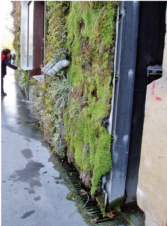
FIGURE 3. The Musée du Quai Branly, in Paris (Project by Jean Nouvel, 2004) is covered by 800 sqm of vertical green. Nutrients for plants are primarily distributed through an irrigation system that cycles water from the top of the system. The continuous flow of water causes extensive wet parts even on the spaces below; for this reason it is necessary to place a water collection grid at the base of the façade. Detail of two felts of reinforced polyamide, containing pipes in the middle for irrigation, a polypropylene geotextile, and the PVC foam that support panels which are fixed to a metal frame is shown.
