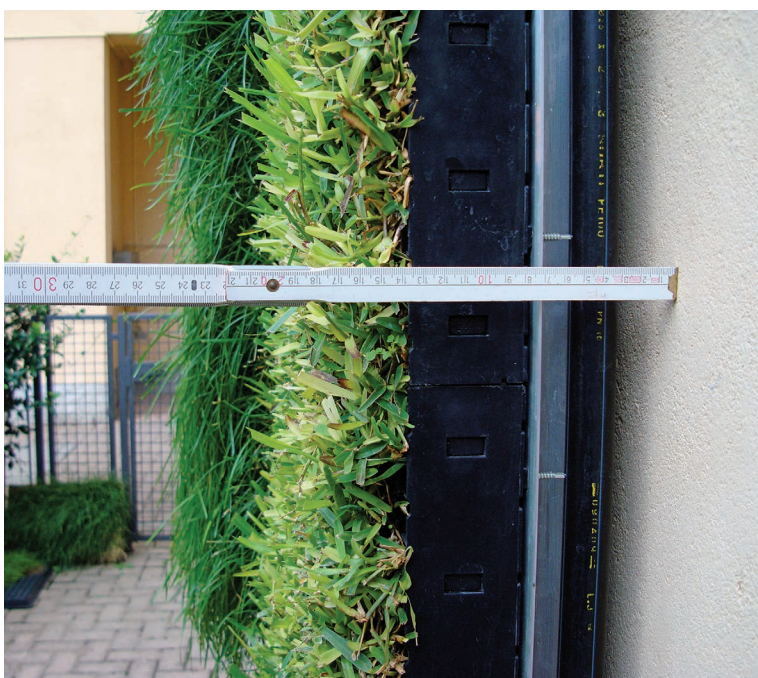
FIGURE 10. The finished façade cladding, depending on the size of the air chamber behind it, is about 130 mm thick.
