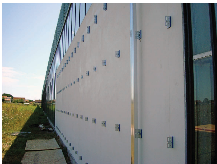
FIGURE 8. Detail of the fixing points of the panels.
