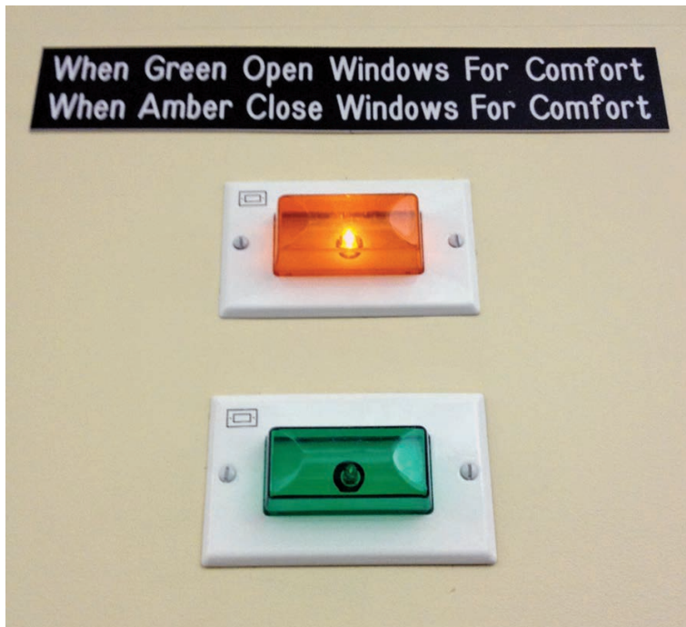
FIGURE 3. Indicator Lights to Engage Building Occupants in Building Energy Management and Personal Comfort Control at UVM George D. Aiken Center. Source: Jodi Smits Anderson, 2014
