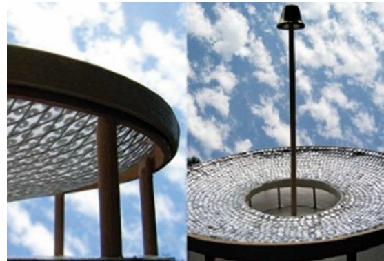
FIGURE 12. Small heliostats on long-span and donut-shape hanging roofs model photos.
