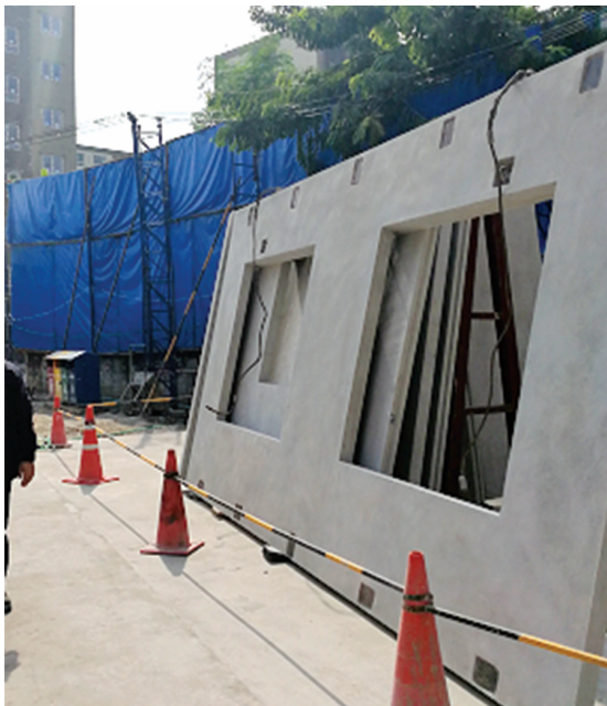
FIGURE 5. Storage of prefabricated wall panels.
