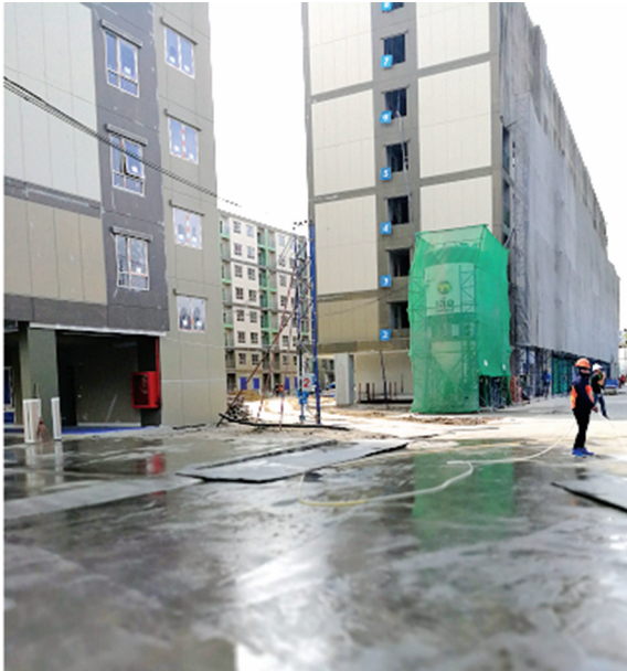
FIGURE 7. Water spray for dust reduction.
