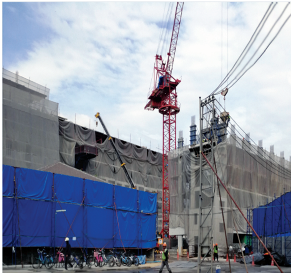
FIGURE 2. Installation of mesh sheets to prevent dust.
