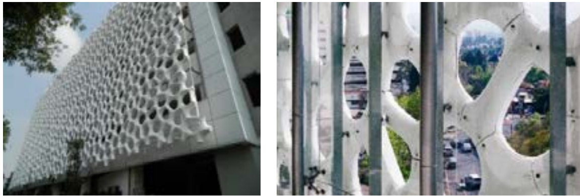
FIGURE 6. [a, b] Mexico City hospital, the Torre de Especialidades Hybrid panels. [c] Energy-Producing Algae Façade which tinted by millions of microscopic algae plants. (14: http://www.archello.com )
