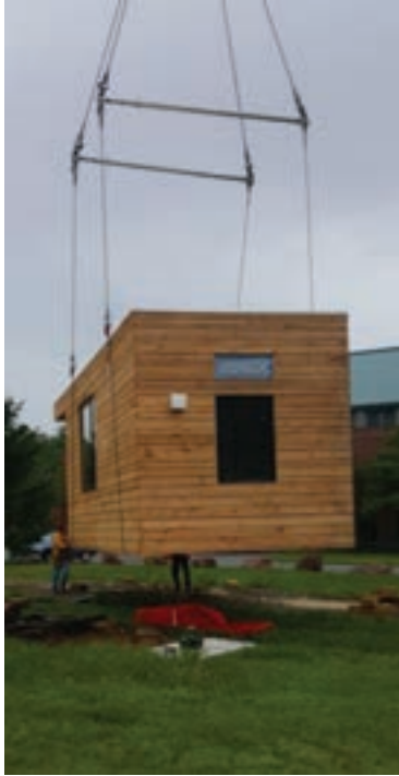
FIGURE 12. SU_CASA being craned onto the trailer.
