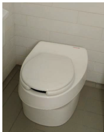
FIGURE 10. The Kern Center uses composting toilets with two Clivus composters located in the basement.
