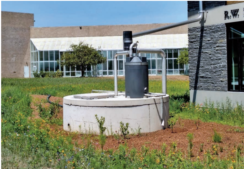
FIGURE 9. Rainwater harvesting collection cistern.
