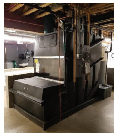
FIGURE 10. The Kern Center uses composting toilets with two Clivus composters located in the basement.
