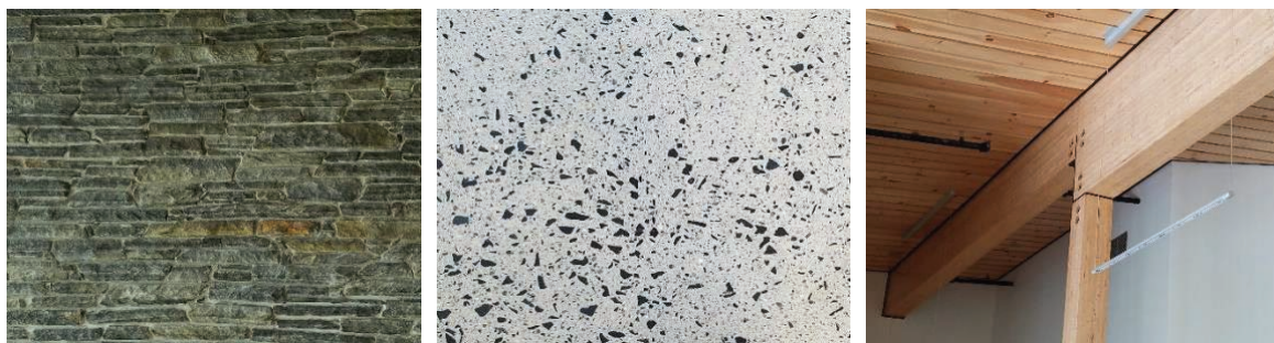
FIGURE 12. Regional materials used in the Kern Center: Ashfield schist for the interior and exterior façade (left) and also featured in the polished concrete floor (center) and laminated Nordic Lam timber framing (right).
