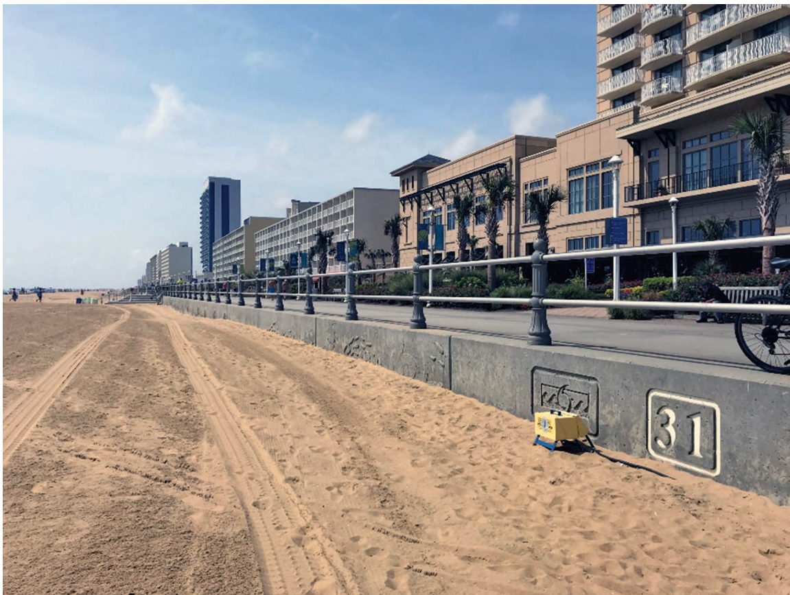
FIGURE 5. The seawall in Virginia Beach, Virginia, built by the Army Corps of Engineers in 2001 also serves as a boardwalk and retains stormwater.
