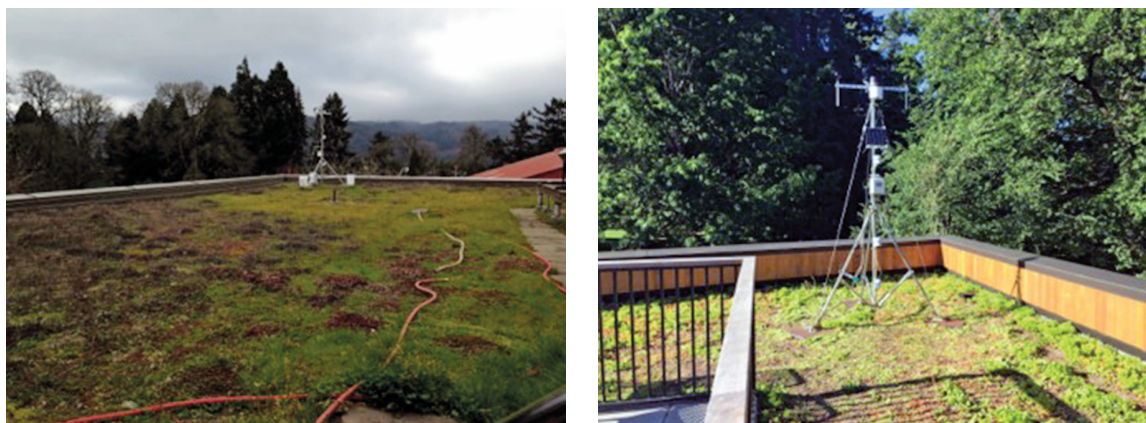
FIGURE 1. Green Roof on (a) Shiley Hall (6 years old) and (b) Templeton Hall (6 months old).
