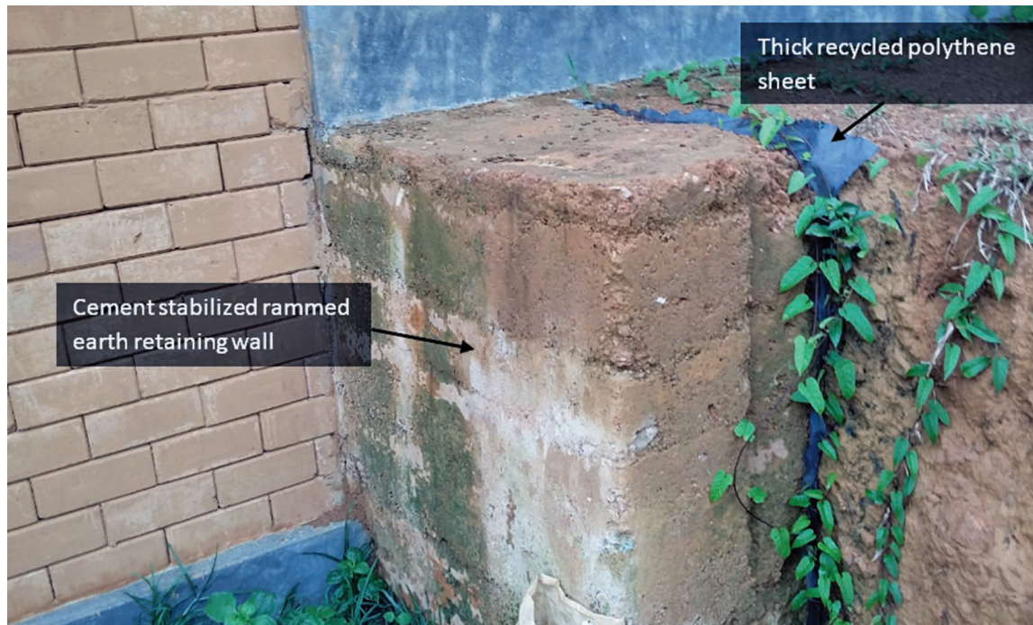
FIGURE 5. A CSRE retaining wall extended beyond the house to retain the soil
