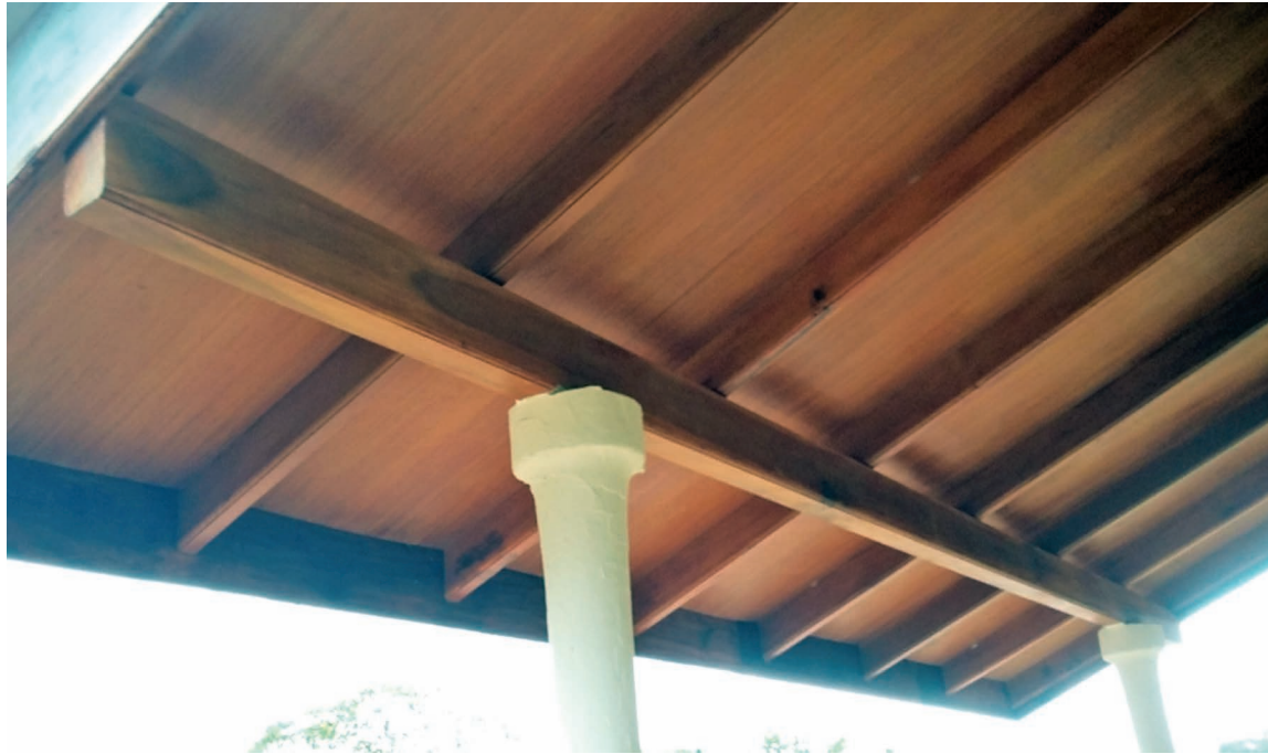
FIGURE 9. Exposed roof structure with the ceiling.
