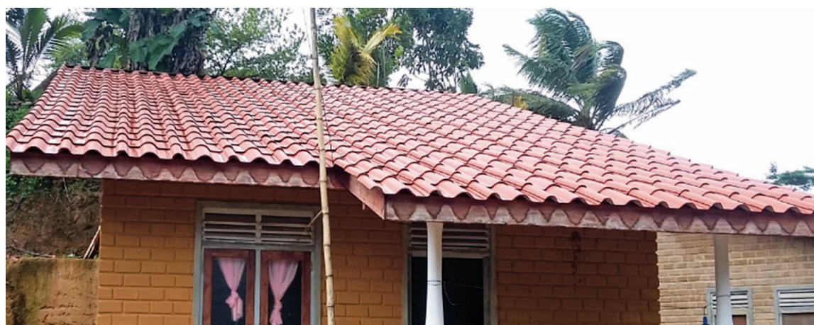
FIGURE 8. Roof with MCR tiles.
