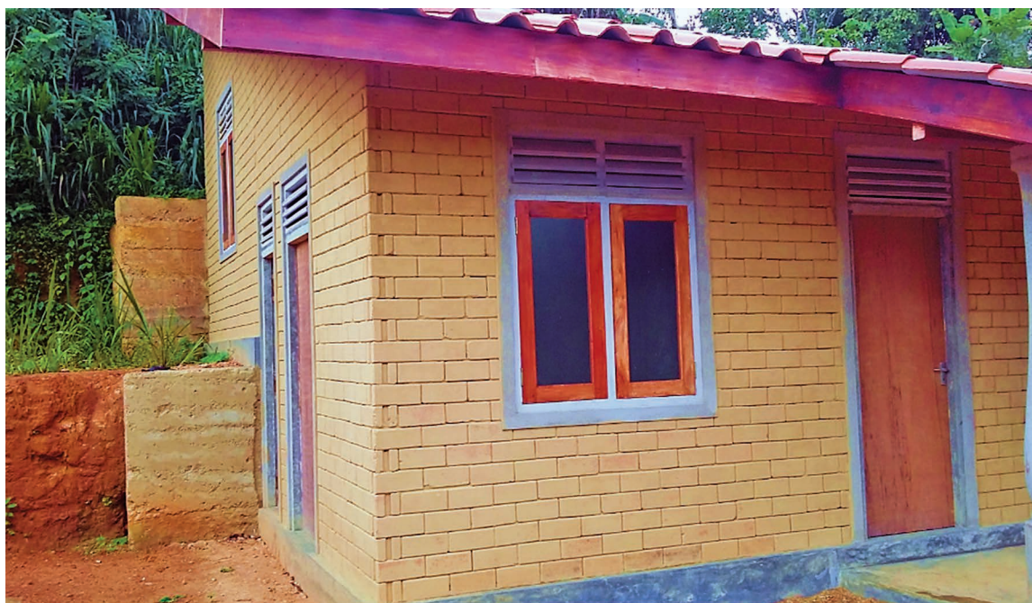
FIGURE 7. Compressed Stabilized Earth Block wall after applying the finishing coat of mud paint.
