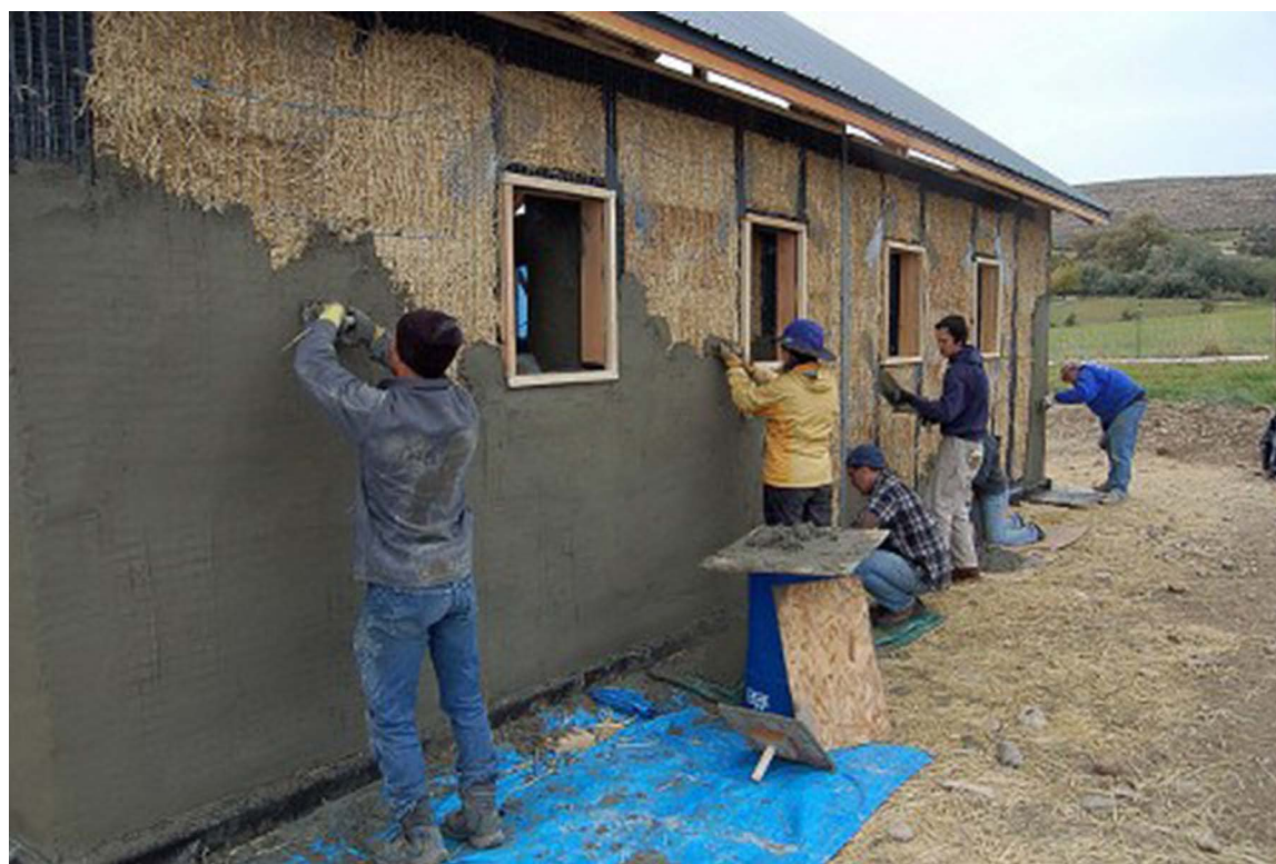
FIGURE 1. Typical straw bale wall (ICFHome, 2017).
