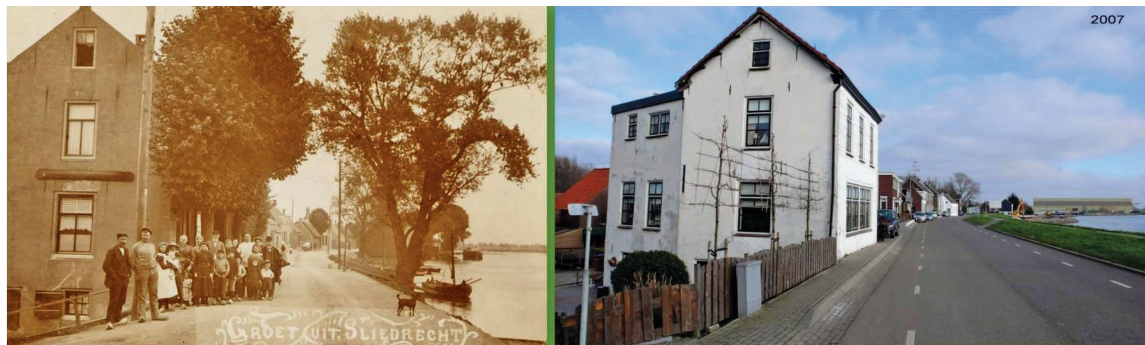
FIGURE 7. On the left a historic photo of the Slidrecht dike, showing the historic presence of trees and buildings in the unbanked area along the river. The trees were removed to accommodate for dike reinforcements, changing the spatial characteristic of the dike ribbon. The picture on the right shows the current situation. Photos: Slidrecht historic society ( http://www.historie-sliedrecht.nl ).
