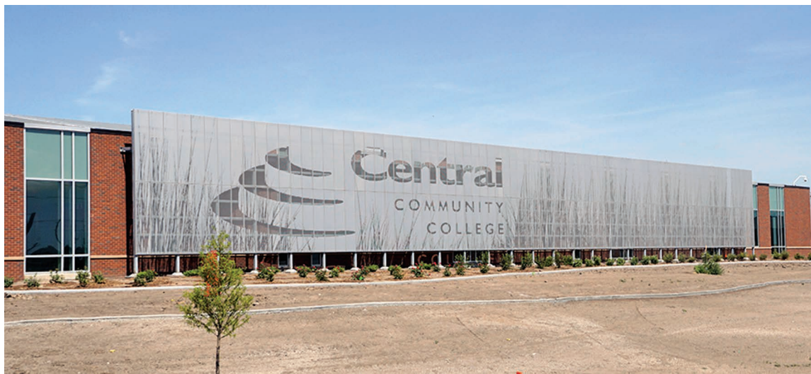
FIGURE 10. Metal scrim that shields the many windows on the south exposure from direct sunlight to eliminate the greenhouse effect. Photo credit—Scott Miller
