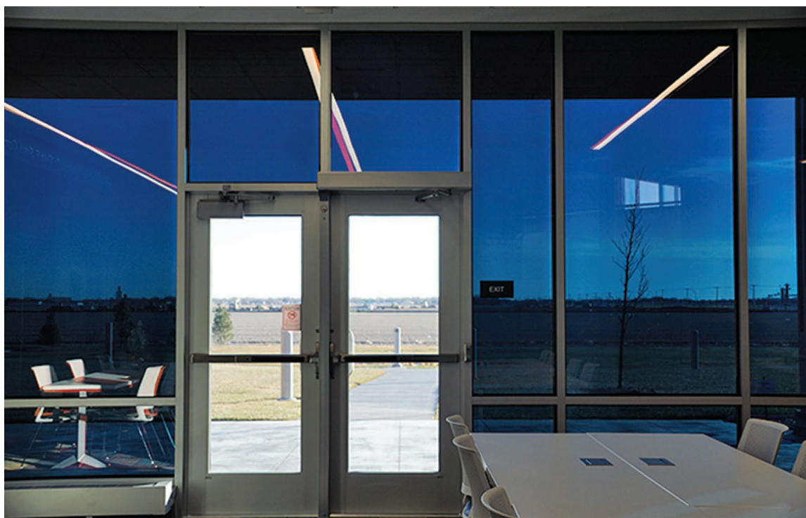
FIGURE 6. Electrochromic windows at the new Kearney Center that allows and blocks natural light. Photo: Scott Miller.
