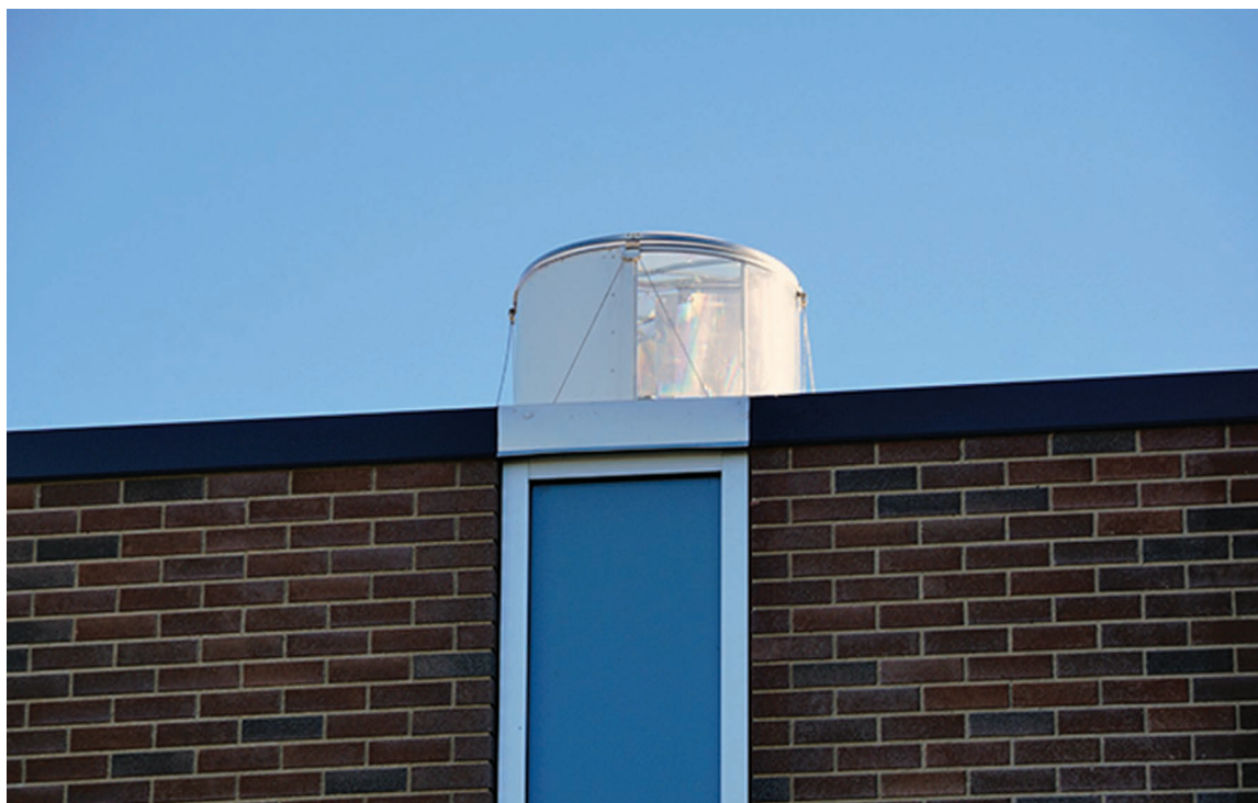
FIGURE 7. Solatube mounted on top of roof. Photo: Scott Miller
