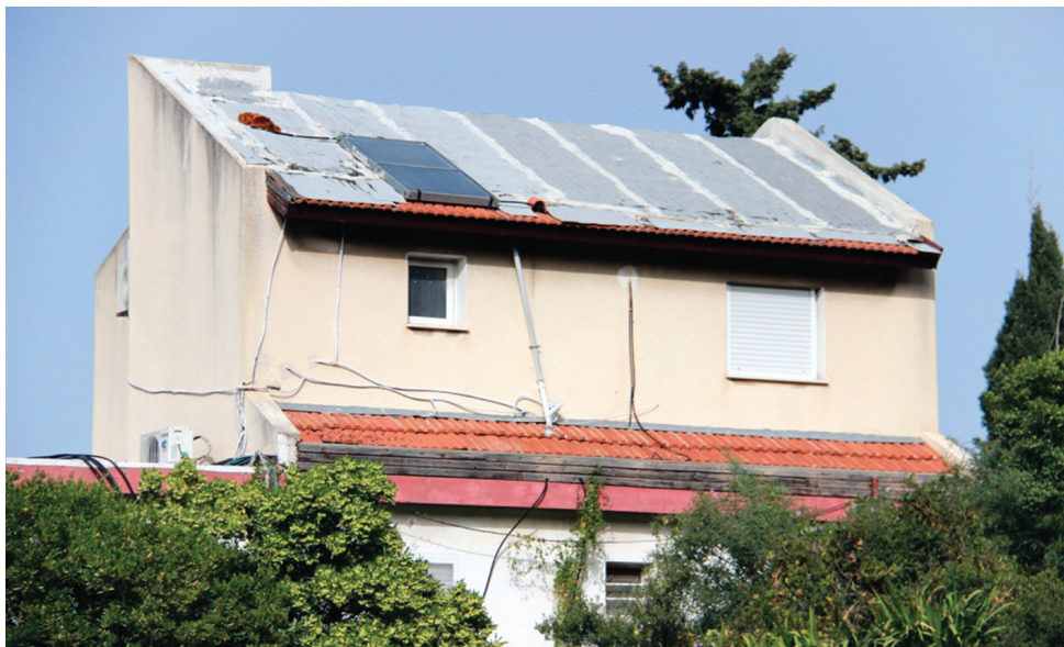
FIGURE 1. Residential house in Nesher, Israel. The roof with red tiles was covered by a white coating by a building’s residents.
