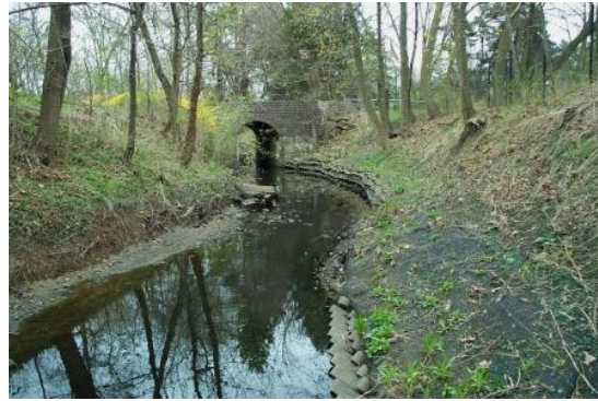
FIGURE 9. A-Jax Stabilization Leading to Erosion of Opposite Banks
