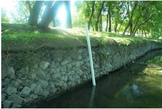
FIGURE 8. Gabions Undermined by Streambed Erosion
