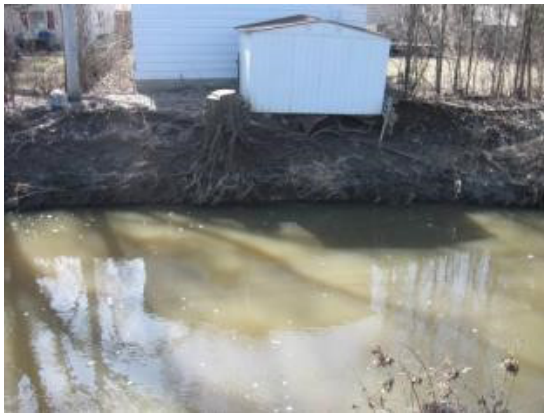
FIGURE 6. Structures Undermined by Streambank Erosion
